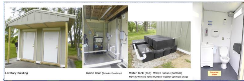
Fig.1 - Golf Course Lavatory Building
