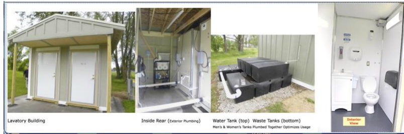
Fig.1 - Golf Course Lavatory Building
