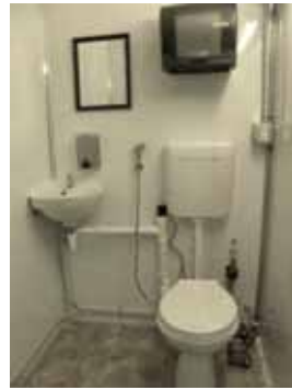
Vinyl Floor - Bidet - Water Pressure Pump
