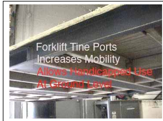
Easy Re-Deployment Steel Frame With Steel Encased Tine Ports
