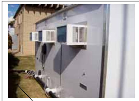
Sewer or Septic Tank Hook-up
